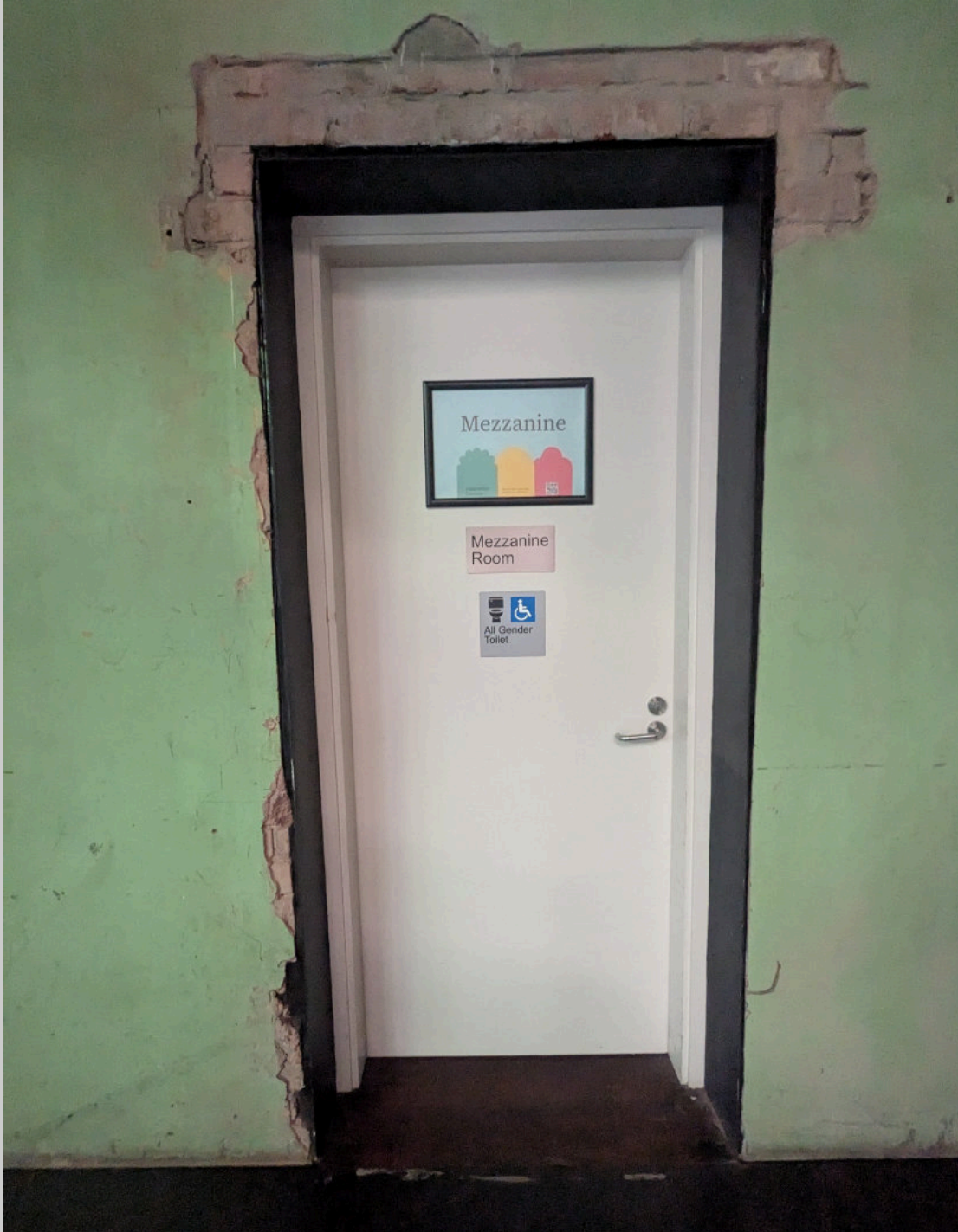
Image Description: A view in front of the white door to the all gender, wheelchair accessible toilet. The walls around it are mint green.
