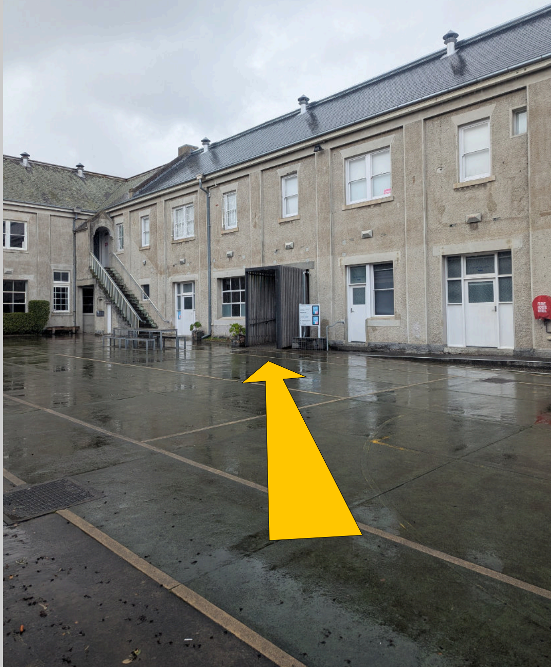
Image Description: A view of the courtyard outside the entrance to the Magdalen Laundry. A graphic Yellow arrow points towards the entrance doorway.
